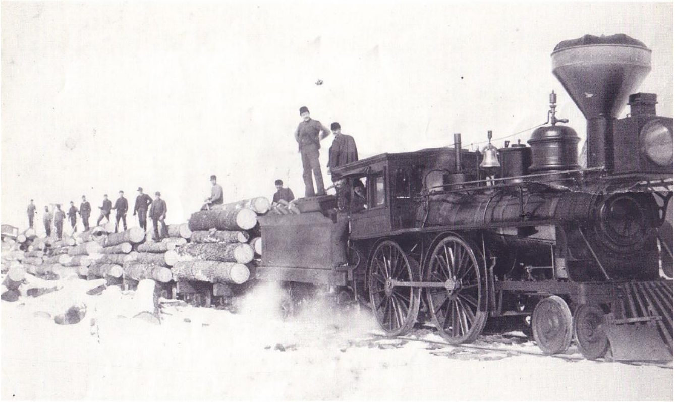
Old "Vanderbilt" was pulling a logging train for the Upham Mfg. Co. in 1890 near Marshfield, Wisconsin. The cylinders and drive rods were inside the frame on this 1847 product of the Taunton Locomotive Works. Ed Upham was the engineer and Frank Welch was the fireman. Courtesy State Historical Society of Wisconsin, Roy L. Martin collection, negative no. WHI M302 11 or WHI M304 96.
