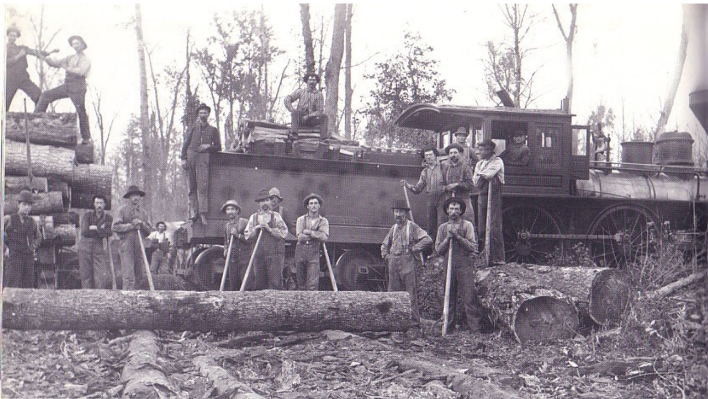
Link and Pin couplers were used on the logging cars and "Old Van" of the Upham railroad, called the Marshfield & Texas. This 1888 photo shows the train at a landing in the woods, possibly on the "Clark County" railroad, with the woods gang posing for the camera. Courtesy State Historical Society of Wisconsin, Roy L. Martin collection.
