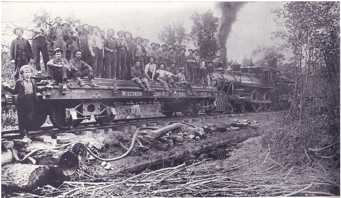
Upham's logging operations north of Athens, Wisconsin were done by rail. Spurs off the Athens – Goodrich mainline were constructed by crews like this one, shown in 1903. No. 1000 was originally Wisconsin Central No. 28. Flat car No. 581 was built in July 1882 by the railroad. It has been "modernized" with new couplers. The stencil on the near end reads, "Williamson & Price, Draw Bar Attachments, Pat'd March 3, 1897." Courtesy State Historical Society of Wisconsin, Copy negative no. WHi (M305) 116.
