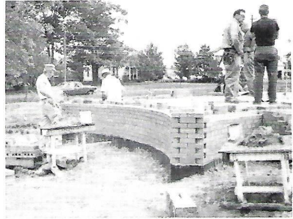
August 9, 1965 Started setting steel I beams. August 17, 1965 Started laying bricks.
