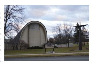
ground on both sides. The apse wall is inverted from tradition, being concave on the outside. The full sanctuary's brick undulating wall flows like a curtain. The church's side walls house rooms for various purposes.
