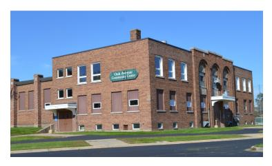
sents strength & stability: made of brick; the north & south sides each having 5 engaged piers with curved copings, raising above the roofline, decorated with a bannered shield. Most original windows have been boarded up, some now contain a small window or glass block.
