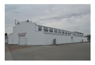
is open beam construction. The "false facades" purposefully hide the low gable roof & side shed roofs behind. The band of large windows along the upper side walls, replaced in c.2015 with vinyl covered wood windows, ensure ample lighting within. This building serves the city not only at Fair time but throughout the year for events, city festivities, etc.
