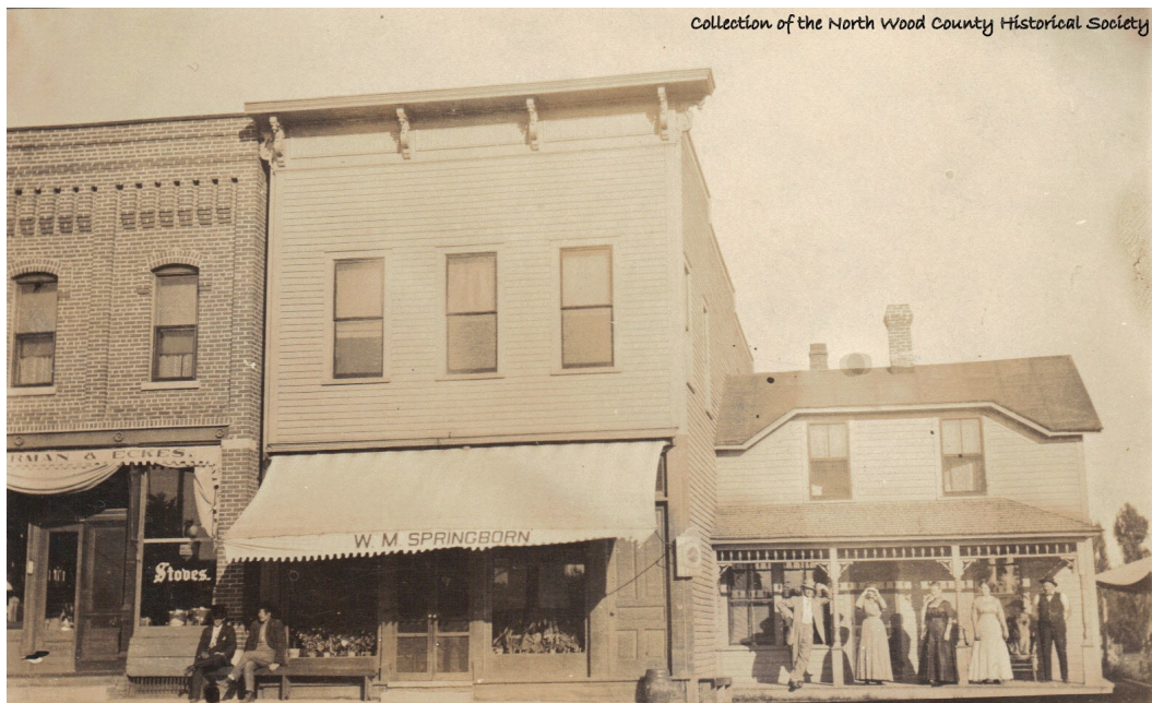
The Eckes Hardware Store is the building on the far left of this picture. Notice the change of building materials used in the buildings. The Eckes Hardware building was built sometime after the Fire of 1887 and was built of brick (as mandated for all new buildings.) The Springborn building in the center of the photo was at the edge of the devastation and not destroyed by the fire.
