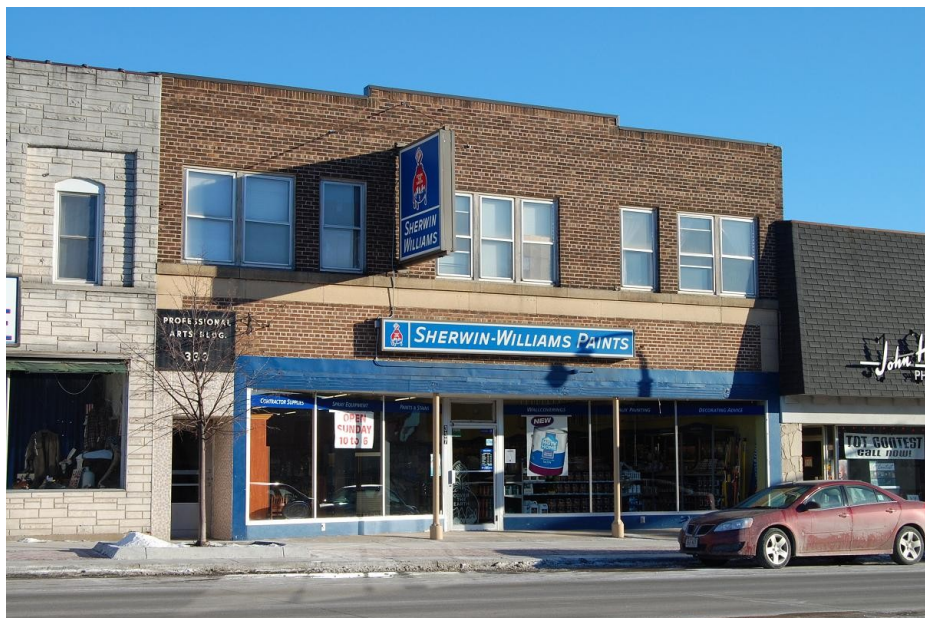
Sherwin Williams Company at 337 South Central Avenue, Spring 2012.
